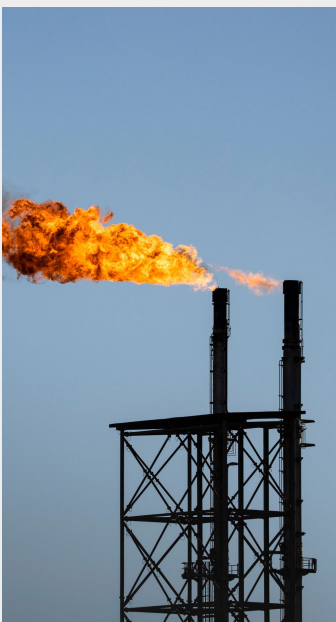
Dampier Pluto Gas Plant in Western Australia © Alex Westover
